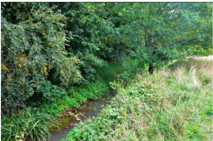
Images 3B and 3P – Method E3 - showing example of accentuating channel narrowing using top of bank spoil (TYPE E3 - only done in upper 200m).
