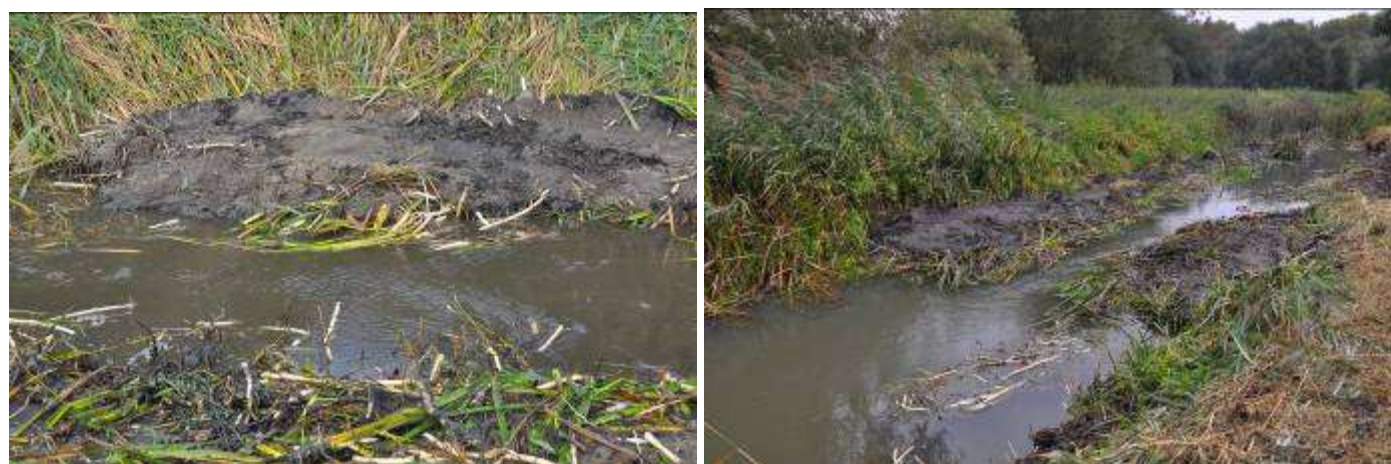
Photos 13PP and 29P. Method C – major narrowing of low-flow channel formed by shoulders on both sides of the channel upstream of pools.
