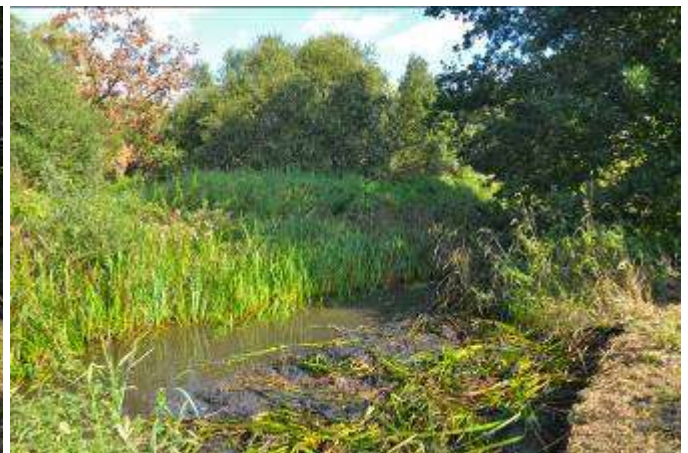
Photos 27B and 27P. Method E1 – major narrowing of low-flow channel formed by shoulder on left bank created using bank re-profile material and reed and silt from a third of the remaining channel (low-flow) width
