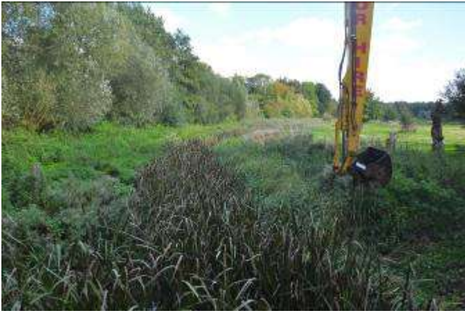
Photos 25B and 25P. Method D – major narrowing of low-flow channel by pushing into the channel a firm sedge fringe and folding in the reed and silt from the far side of the channel into void created behind the sedge fringe and the rest of the bank
