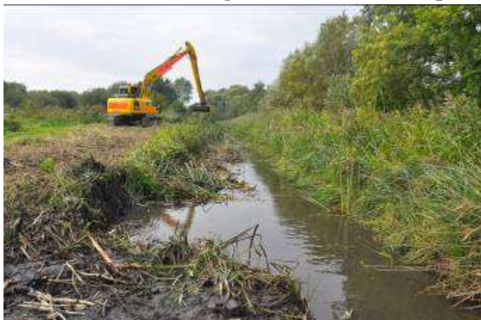
Image 14P & 28P – Method F1 – pool with vertical water vole edge
