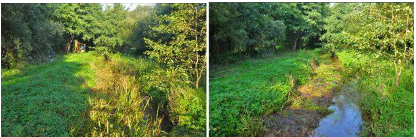
Photos 9B (Before) and 9P (Post) – Method A – simple folding of reed and silt from one side the channel to the other.
