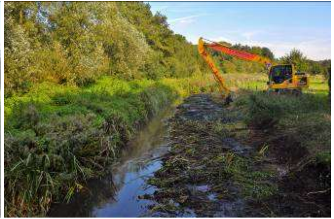
Photos 25B and 25P. Method D – major narrowing of low-flow channel by pushing into the channel a firm sedge fringe and folding in the reed and silt from the far side of the channel into void created behind the sedge fringe and the rest of the bank
