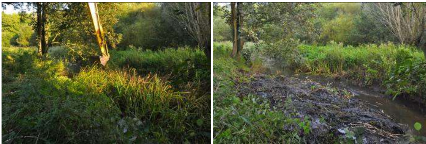
Photos 11B and 11P – Method A – simple folding of reed and silt from far side of the channel to the near side.
