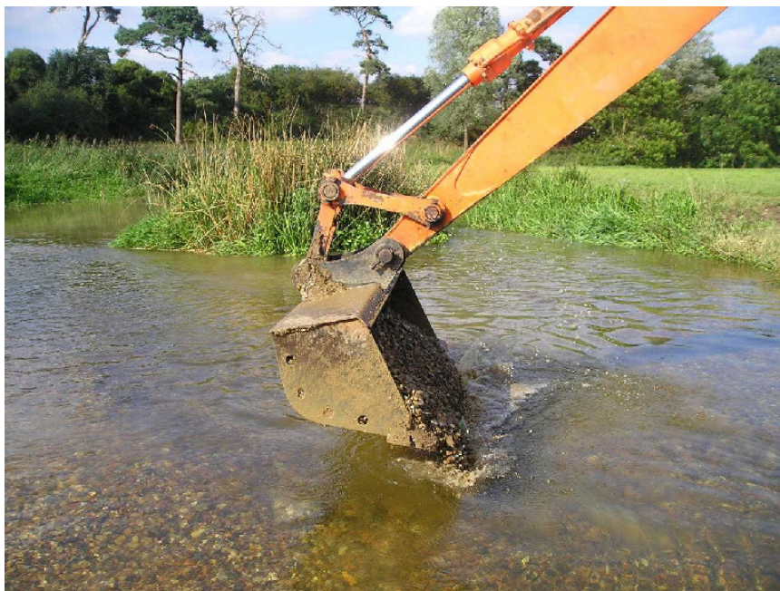
Photo 9. Placing of gravel, Flixton
