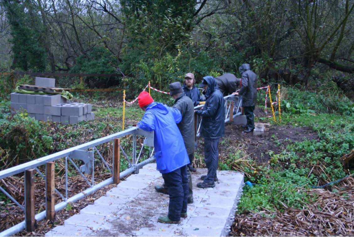
2 Manhandling the first truss across the river
