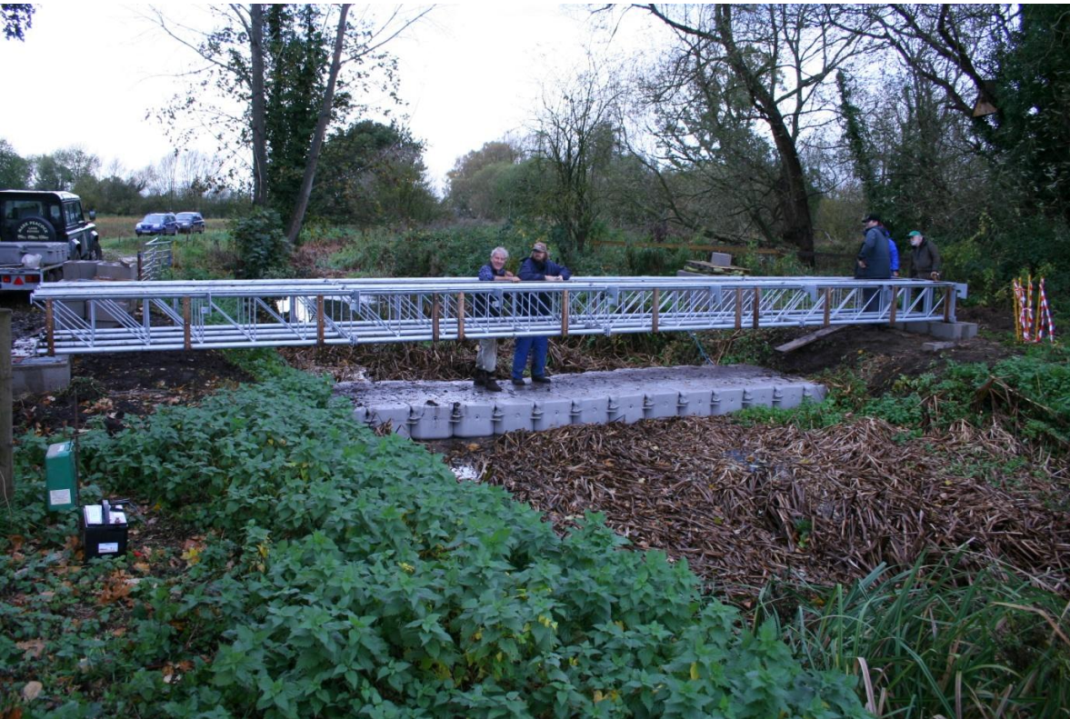
3 The bridge takes shape
