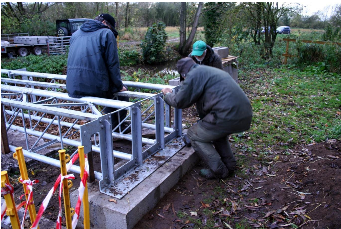
5 Fixing the bridge to it's anchor points
