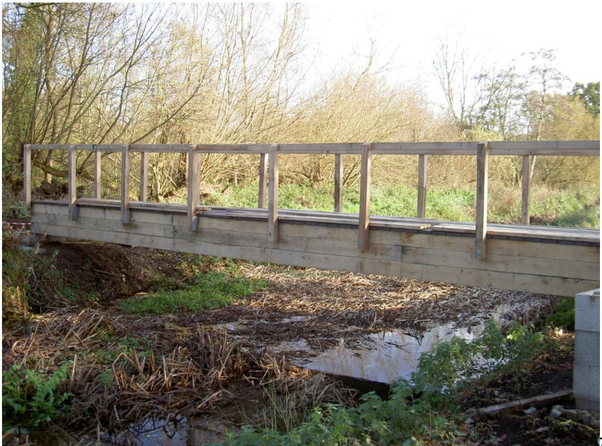
The finishing touches – decking and handrails
